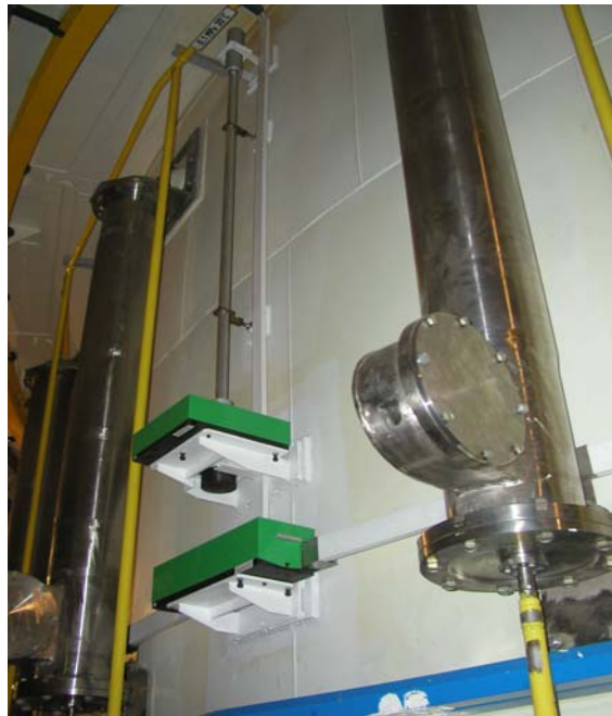
Fig . 4. The installation of hydrolevelling and pendometric sensors on the reactor shaft.
