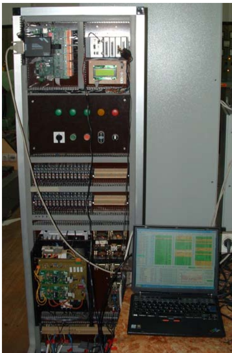
Fig.7. Digital control system
