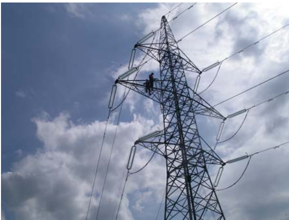
Fig.10. Conductor arrangement on the 49 th tower
