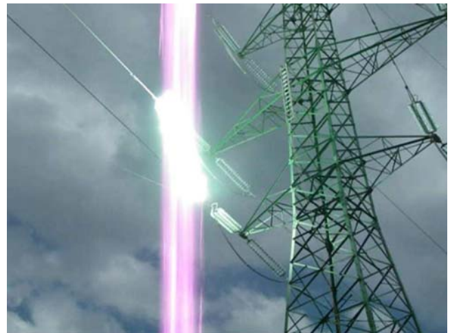
Fig.13. Arc flashing during L1-L2 fault testing
