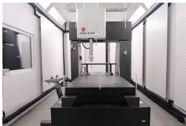
Fig.3. Leitz PMM 12106 machine placed in the laboratory air-conditioned using water panels and controlled air flow.
